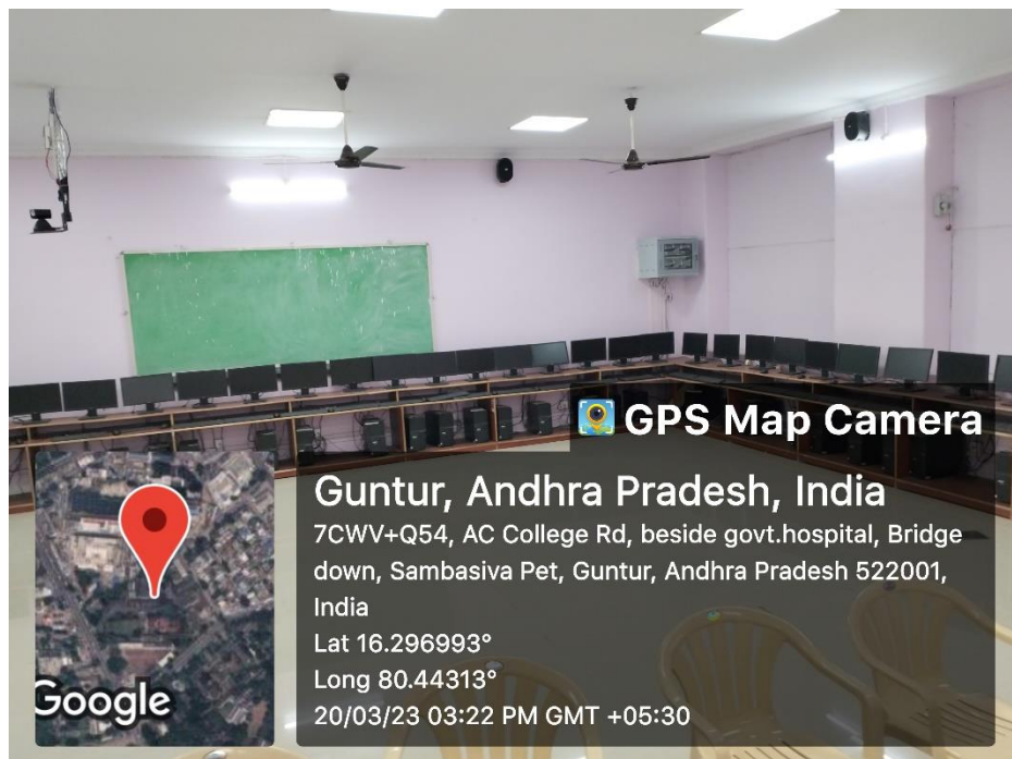
LED Bulbs in RUSA Lab
